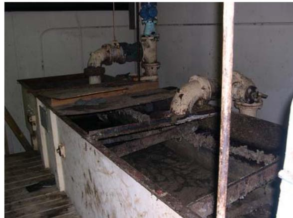
Plant staff is pleased with the operation of the scum concentrators. The scum concentrators need only routine maintenance, and very infrequently is it necessary to replace the scum collector chain and flights. In addition to the scum concentrators significantly lowering handling and problematic disposal costs by reducing scum weight and volume, the concentrated scum is a highly effective supplemental fuel for the incinerator, reducing the demand for fuel oil.
