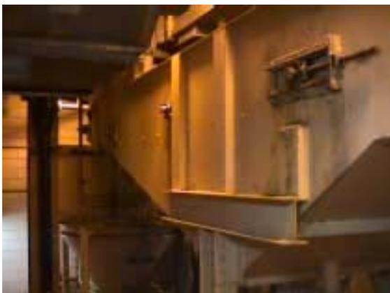
Two scum concentrators were installed in 1976 and each scum concentration tank had nominal dimensions of 4' wide x 18' long x 5' deep, providing a nominal water surface area of 50 square feet and a nominal working volume of 600 gallons. Each tank was designed for 100 gpm of blended scum flow. Each tank was fabricated from 1/4" minimum thickness carbon steel and discharged scum to a mixed and heated holding tank. The scum collector chain was malleable iron and the flights were redwood.
